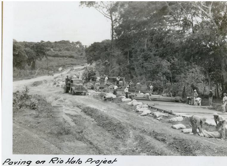
Paving on Rio Hato Project, 21 May 1942 (John L Humbard)
