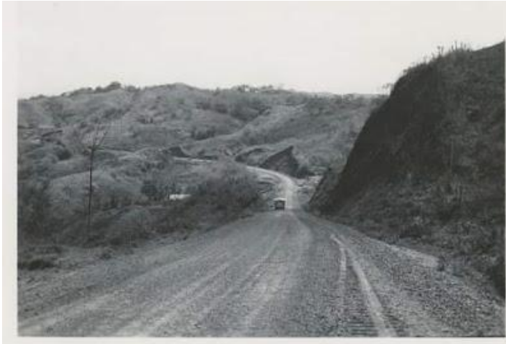
Photograph from 1942 showing the progress of the civil works for Transisthmian Highway
