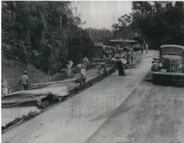
Pan-American Highway under construction in 1942
