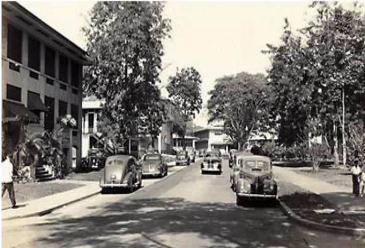
Another pre-switch photograph showing traffic parked on the left.
