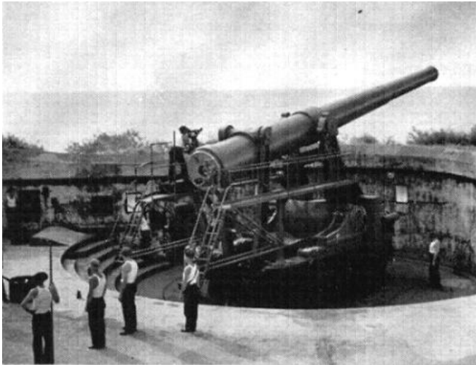
A “disappearing” 14-inch coastal artillery gun, 25 years old in 1941, probably at Battery Warren on Flamenco Island. The gun had a range of 13.64 miles. Beneath each were a powder magazine and shell store. A lift descended 250-feet to a shoreline railway siding tunnel
