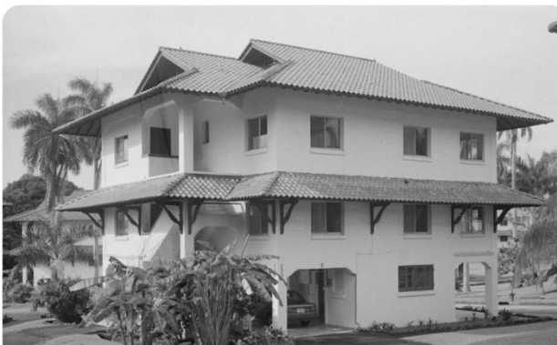
NCO housing at Albrook
