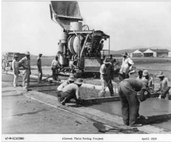
Laying concrete paving at Albrook Field in April 1939 41
