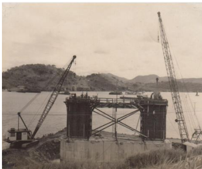
The bridge bases under construction
