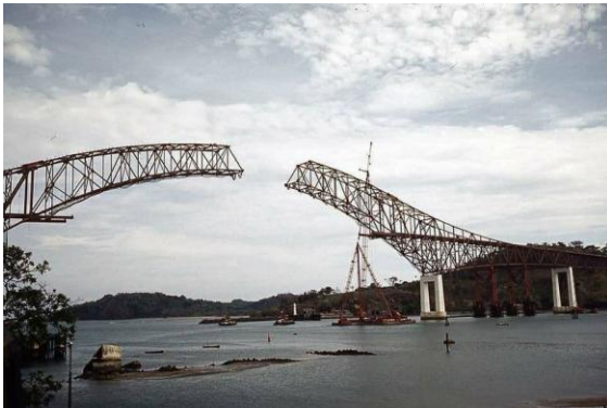
The bridge under construction in 1961
