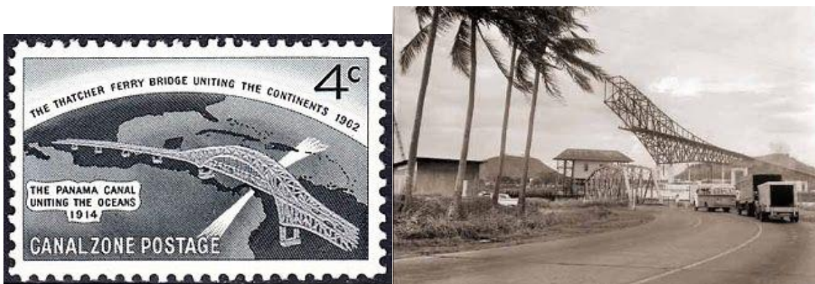
Commemorative stamp and the "Bridge of the Americas" under construction
