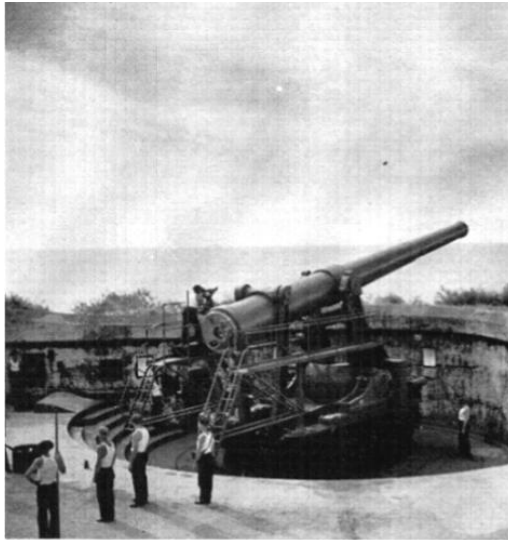
14-inch gun on a “disappearing” mount. There were 7 of these guns 13
