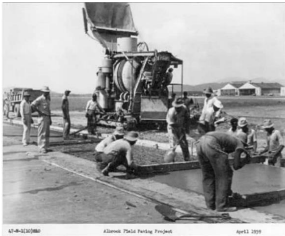
Laying concrete paving at Albrook Field in April 1939 37
